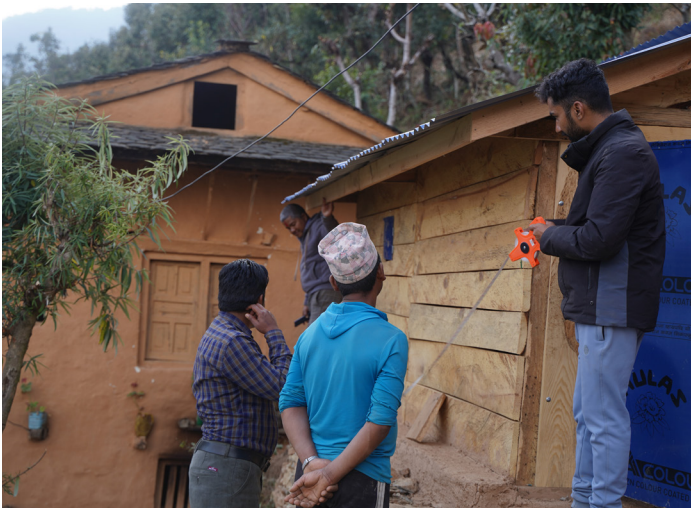
An engineer monitoring the newly built temporary shelter. ©Plan International
